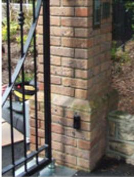
Photograph 1: Brick Pillars - Corbelled brick pillar increasing gap size
