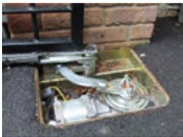
Photograph 2: Gate & Motor Arm - Spine of gate sat forward of mounting pin on motor, increasing gap size and creating a crushing hazard
